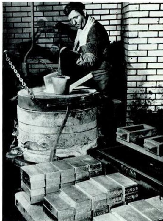
**This is a foreign "melt."** Gold from overseas arrives in bricks of varying sizes, must be melted down and made up into the standard bars you see opposite. This furnace is a big one. It melts 10,000 ounces of gold at one time. Its temperature must be 2,000° Fahrenheit. At a lower temperature gold will not pour properly, at a higher one too much will go off in smoke and fumes.
